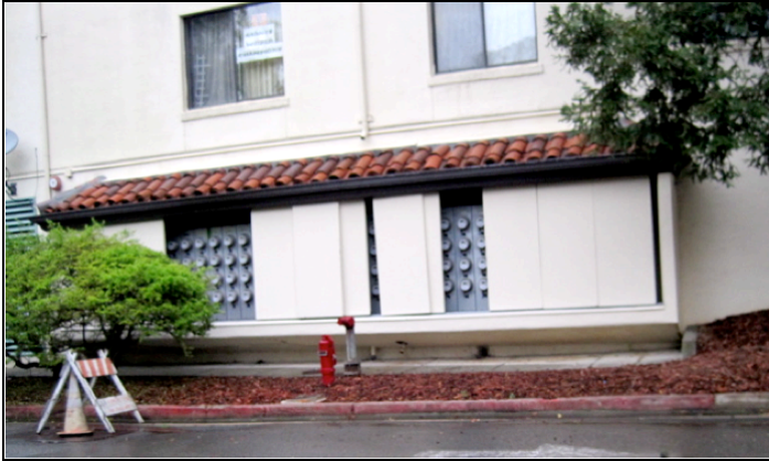
112 Smart Meters in apartment complex
